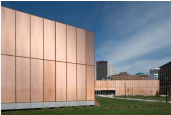
Des Moines Library, USA. Encapsulated expanded metal within glass to achieve this stunning Day/Night effect.
